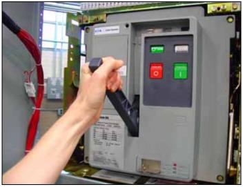
Figure 23. Pumping Handle Charges Stored Energy Mechanism (Closed Transition Shown).
